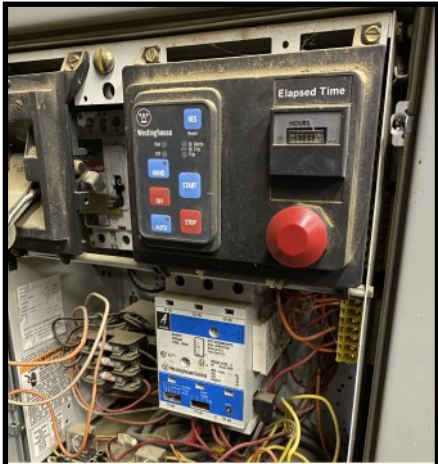
Existing irrigation pump motor control center (MCC) with constant-speed motor starter, manual controls, and mechanical pressure regulation. Proposed upgrade will integrate a variable frequency drive (VFD) to provide modern variable-speed pump control and improved energy efficiency
